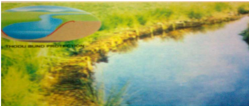
Thodu bund with coir netting
